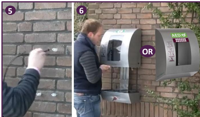
5. Push power cable through the hole 6. Open cabinet and install it on the dowel screws
